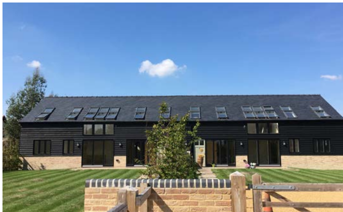
Figure 106: Terraced housing in Haslingfield
