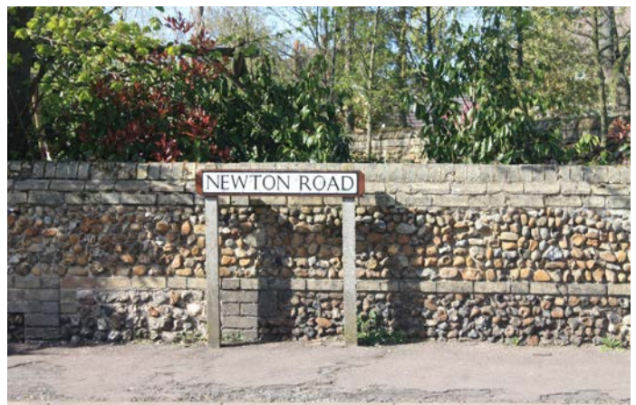
Figure 78: Number 2 boundary wall
