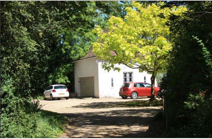
Figure 70: Kings Farmhouse Dovecote, 21 High Street.
