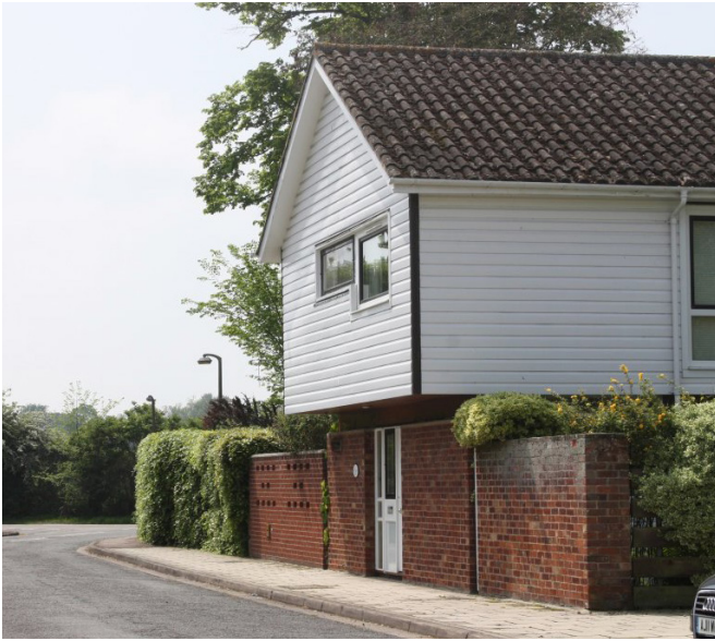
Figure 18: 1 Courtyards, Whittlesford Road
