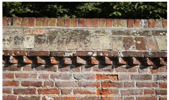
Figure 77: Boundary wall. The Manor House, Bridge Lane.
