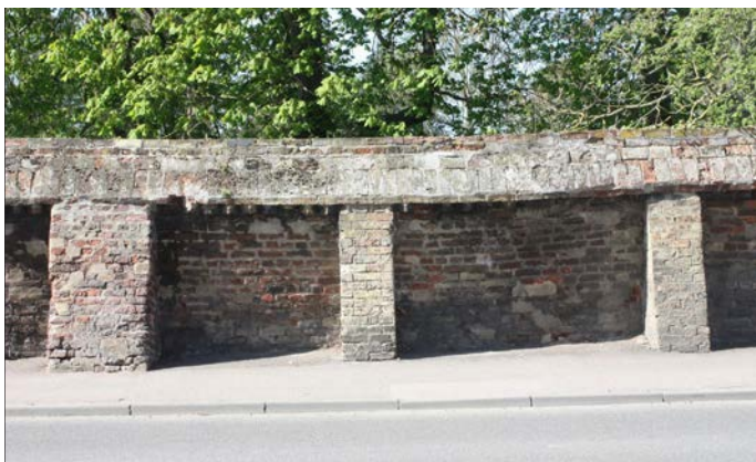
Figure 75: Boundary wall. The Manor House, Bridge Lane.
