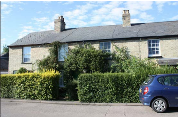
Figure 67: Terrace, 21-27 Hauxton Road.
