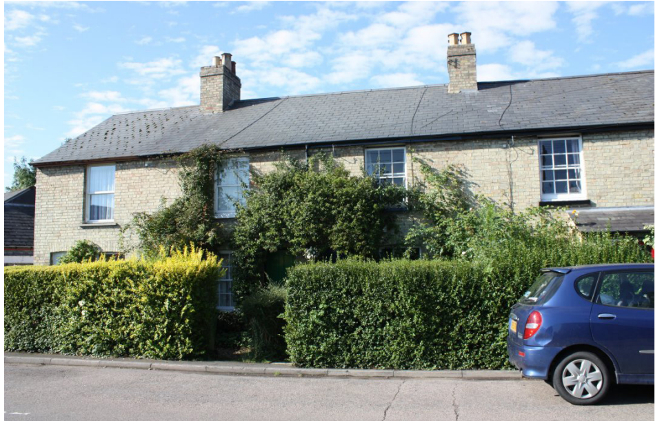
Figure 51: Victorian Terrace, 21-27 Hauxton Road
