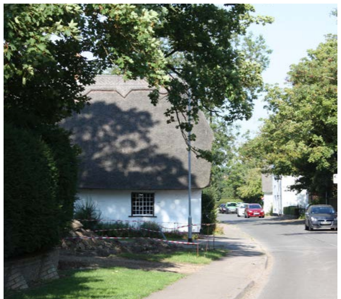
Figure 26: White's Farm House, 26 High Street
